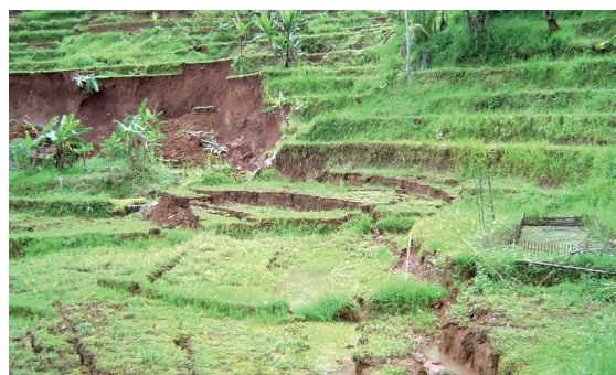
Crown of landslide height 3 m as a rice field at Situmandala village, Ciamis, West Java.
