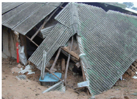
<Damaged House by Landslide in 2003> - Samcheok City, Gangwon Province -
